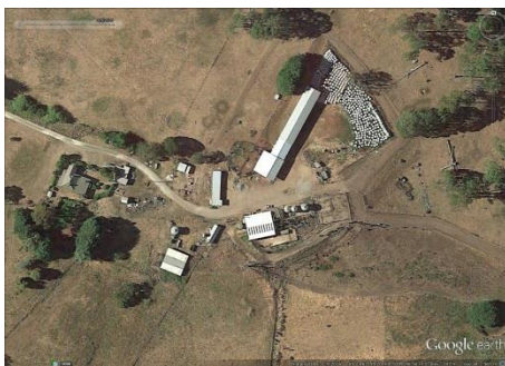
Figure 6. 5.2.1 Dairy sheds and yards
